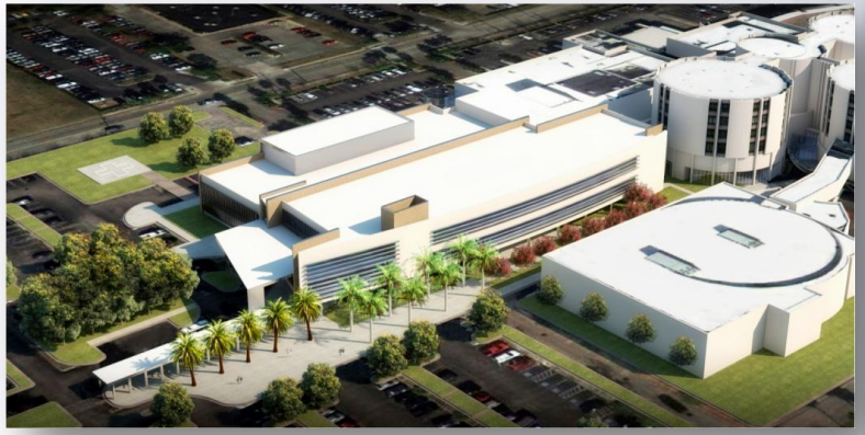
Clear Lake Regional Medical Center - $92 M expansion is complete
