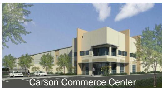
Carson Commerce Center Pasadena, TX – SH 225 22-acre development. 365,000 SF build-out. Under construction.
