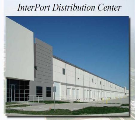
InterPort Distribution Center Bayport Industrial District – Bay Area Blvd. 90-acre development. 1.3 million SF build-out. 296,400 SF available
